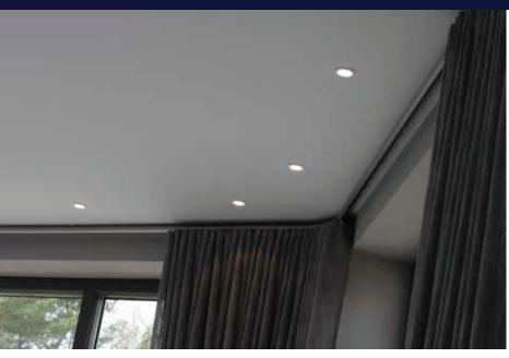
Textured White or Black pinspot with small trim. The LED chip is recessed back into the fitting reducing glare. Scallop effect is created when placed close to a wall. Coloured LED is also available.
